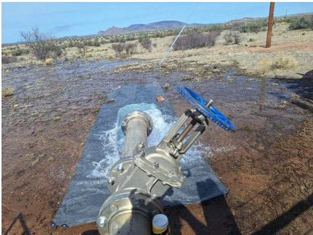
PHOTO 3 (2/23/24): Aquifer testing at 395 gallons per minute (facing north).
