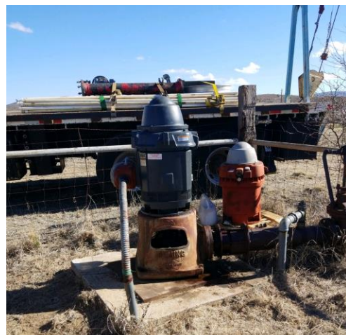
PHOTO 4 (3/1/24): Well head placed back into its original configuration (facing south).
